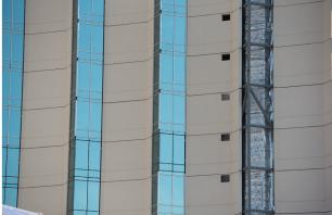
To assure PCL that the prefabricated approach would provide the same quality as field applied EIFS, yet in a fraction of the time, Swanson & Youngdale worked with the Lutz Company to develop a full section of exterior cladding with an integrated window system. After seeing the Outsulite<sup>™</sup> Tech21 wall section, PCL was convinced. The completed section was then shown to the Design Team and Owner, both of whom signed off on the accelerated construction approach.
